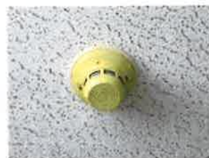
Photo: Smoke Detector (Unknown manufacture)
