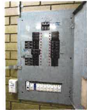
Photos: Curves Switchboard
