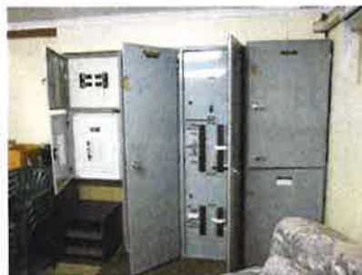
Photo: Main Switchboard
