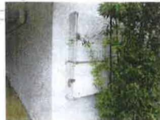
Photo: Outdoor Metering Enclosure
