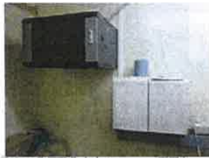
Photo: Building Occupant Warning System (Black cabinet)
