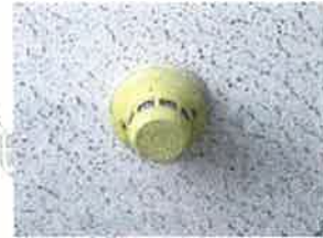
Photo: Smoke Detector (Unknown manufacture)
