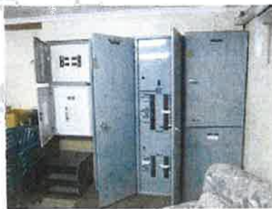
Photo: Main Switchboard
