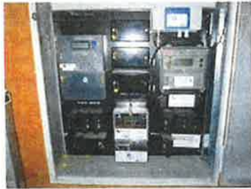
Photo: Main Switchboard with Metering
