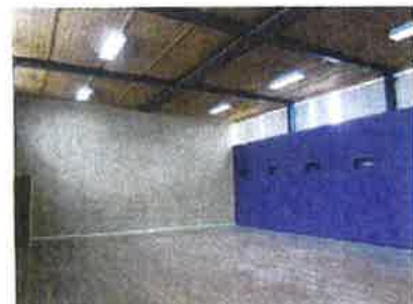
Photo: Main Hall Lighting
