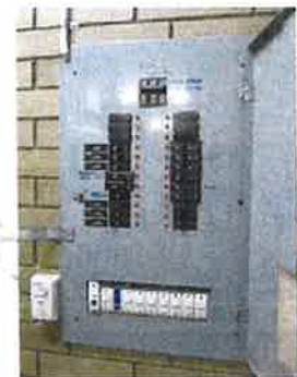
Photos: Curves Switchboard
