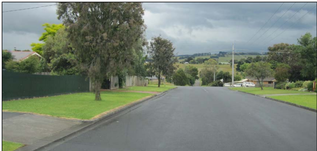
WORTHY STREET LOOKING WEST TOWARDS BROWN STREET
