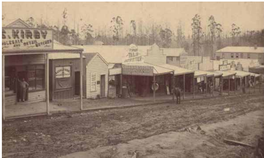
Historical photograph of Commercial Street
