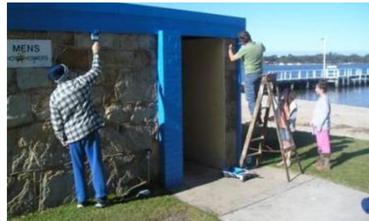
Photo source: Village Well website – Volunteers painting the toilet block
