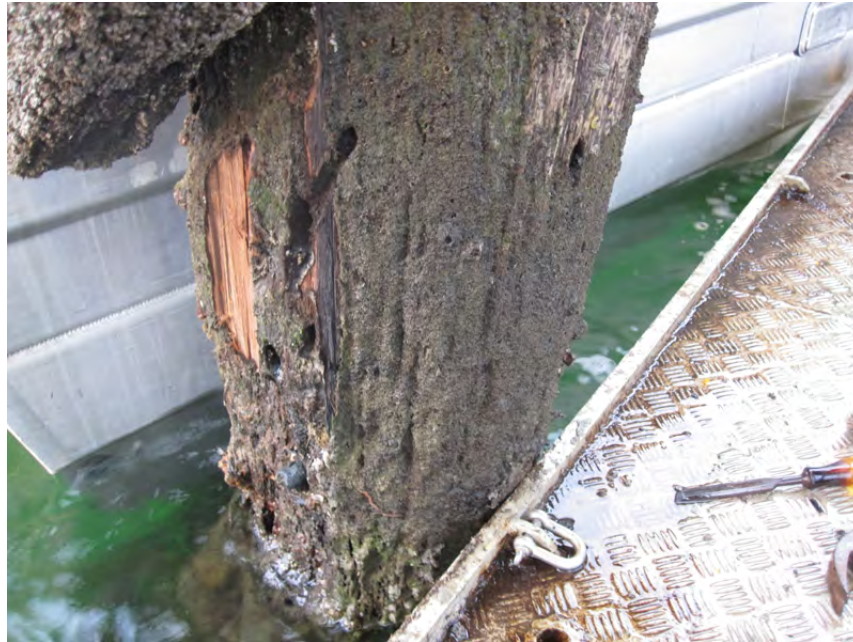
Figure 14: Pile 239B, low tide region showing flattened (checked) face for cross-brace now lost, and projecting end of bolt visible above waterline. Light teredinid attack, freshly chiseled area without teredinid damage.
