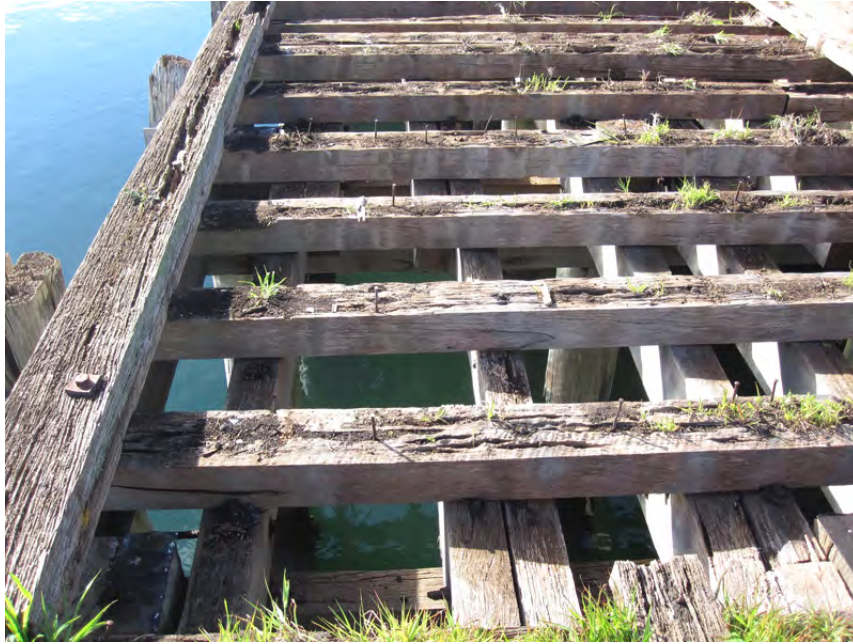
Figure 26: Area 5, transom resting on longitudinal beams resting on crossheads.
