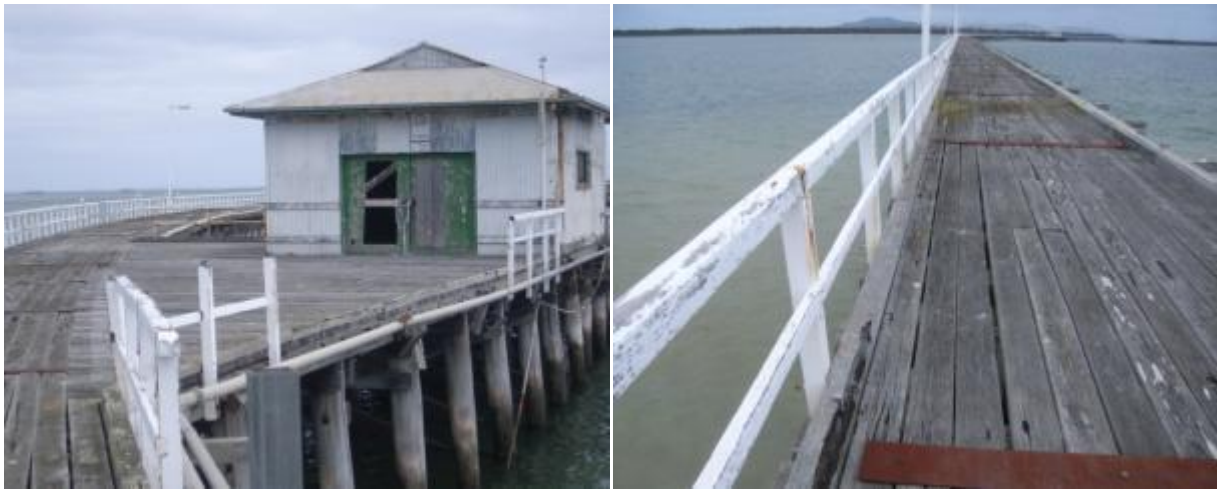
Figures F12-13: Timber handrails
