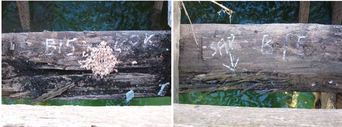
Figure 20: Longitudinal beam 15. Left photo shows streak of decay 15 mm wide, adjacent drilled timber (note shavings) sound. Right photo showing wane and sapwood edge lost or decayed/breaking away.
