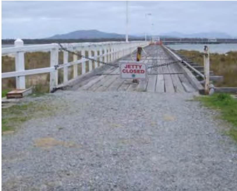
Figure F11: Access to the start of the Jetty
