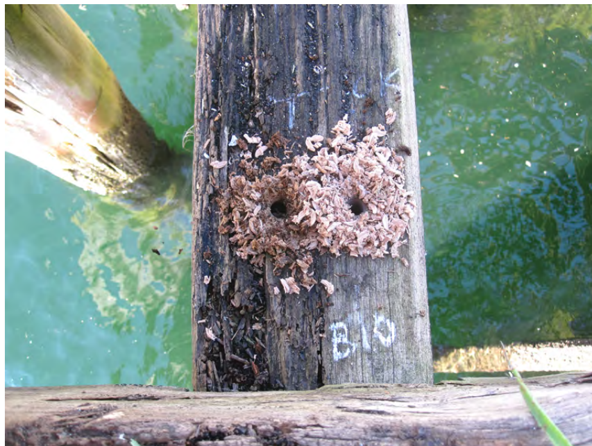
Figure 18: Longitudinal beam 10 over crosshead 279A showing left side of beam damaged by termites and decay (dark coloured shavings) and right side of beam sound (light coloured shavings).
