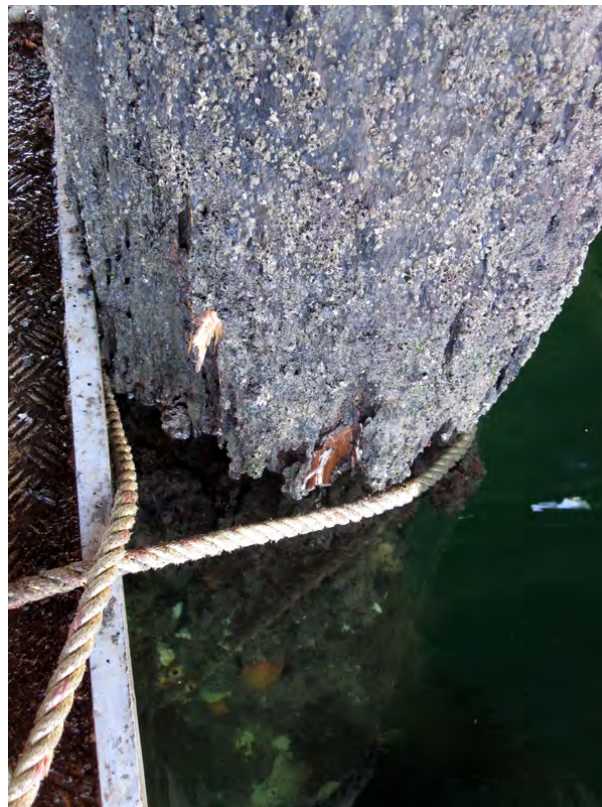
Figure 21: Pile 296A, with only 100-120 mm sound wood remaining. Freshly chiseled region near rope showing some white calcareous-lined teredinid tunnels.
