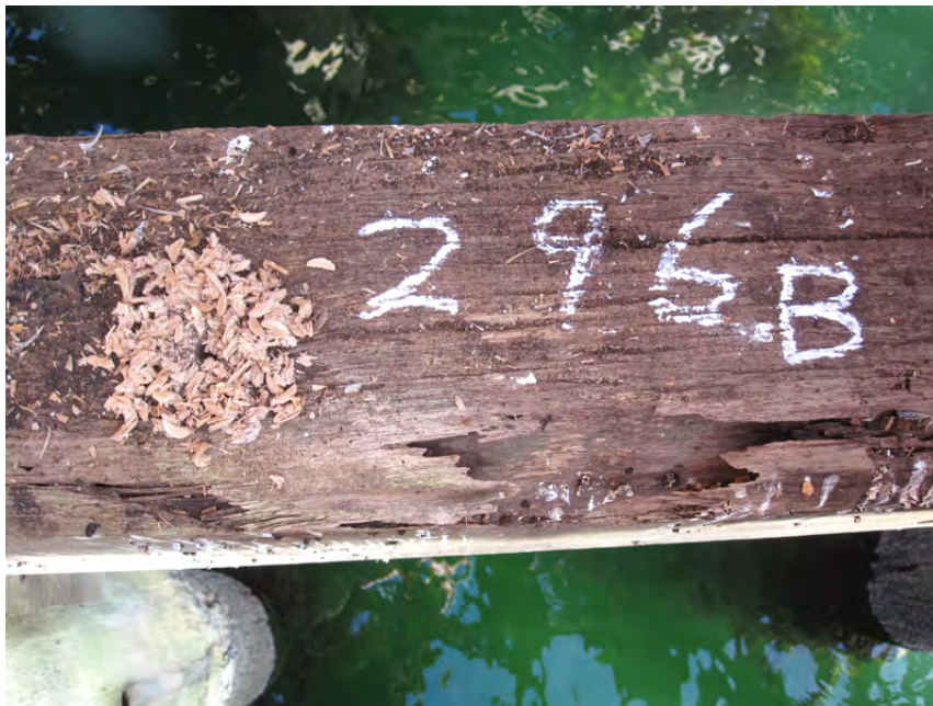
Figure 28: Crosshead above 296B pile, showing sapwood edge lost to decay (lower edge in photo) and drill shavings 20 mm in from sapwood edge indicating heartwood is sound.
