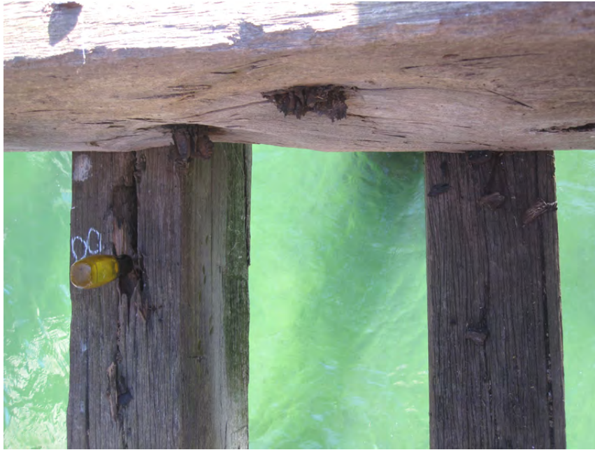
Figure 5: Southern side crosshead (left) hollowed by termites. Northern side crosshead (right) with moderate termite damage, heavier damage other end.
