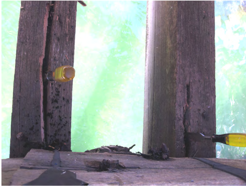
Figure 4: Northern side crosshead (left) with 120 mm deep crevice of termite damage. Southern side crosshead (right) with moderate termite damage at one end.
