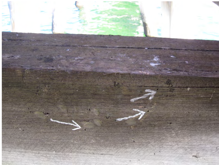
Figure 3: Side of crosshead with minor borer damage caused before the log was sawn, of no concern.
