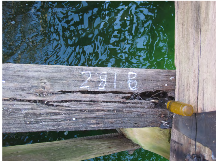
Figure 17: Crosshead 281B with termite damage 600 mm along end of beam.
