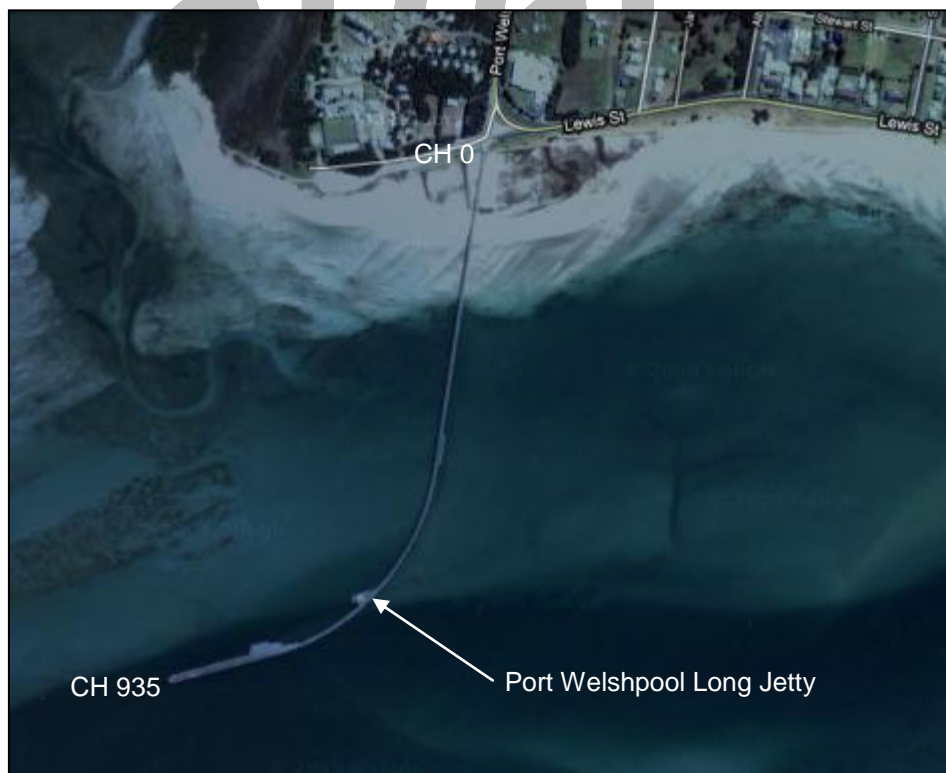
Figure 2.1.2: Port Welshpool Long Jetty Aerial View and Location Plan (Image courtesy of Google Maps)
