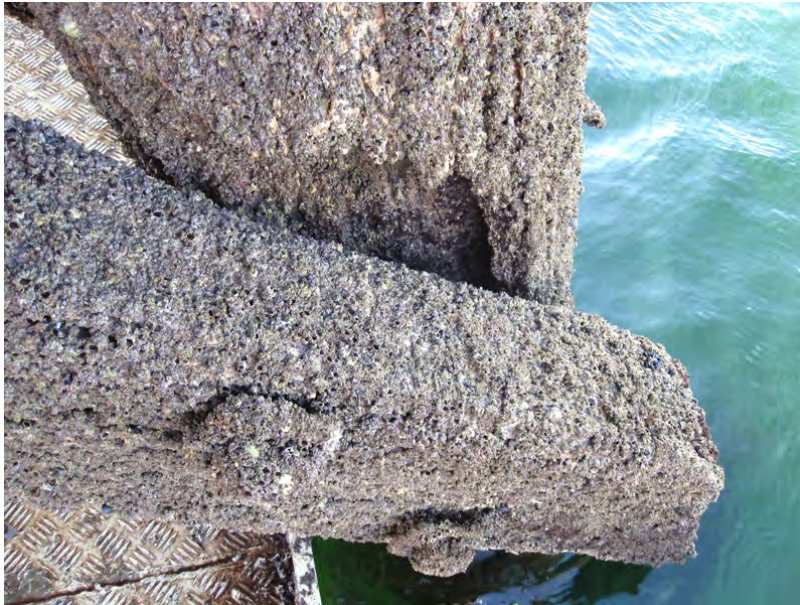
Figure 6: Pile 232B, showing mid-tide region with erosion caused by Limnoria behind cross-brace.
