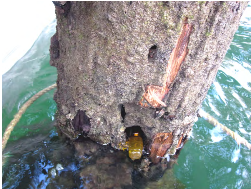
Figure 10: Pile 237B, low tide region showing chisel in one of the 50 mm diameter bolt holes, pile unserviceable.
