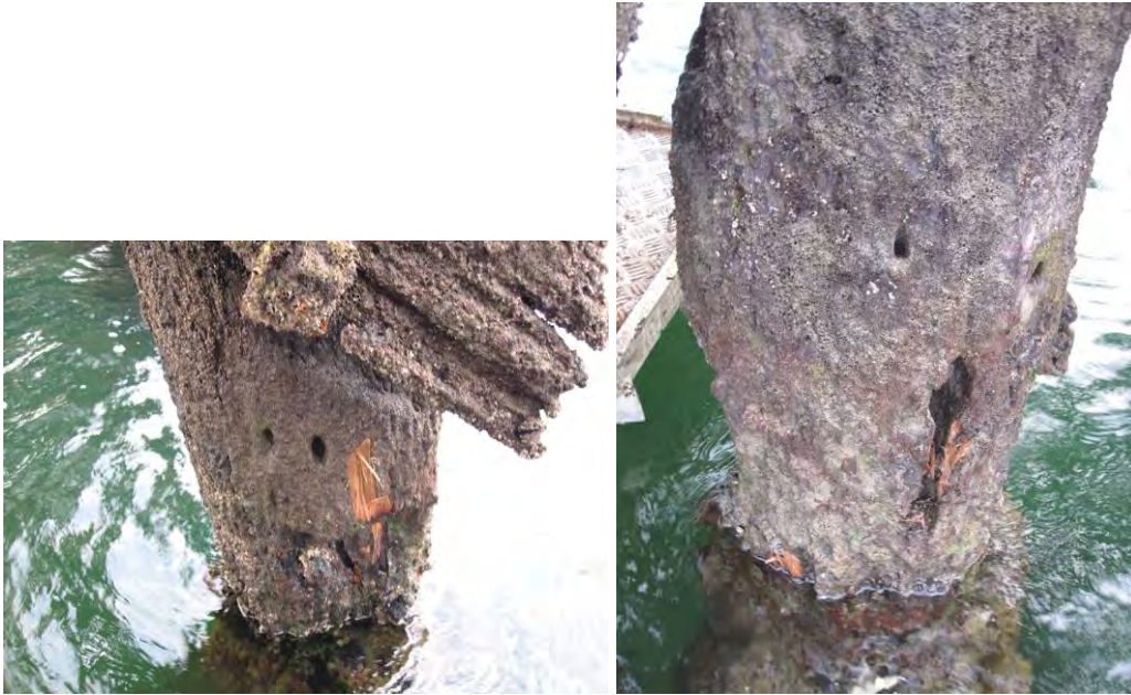
Figure 12: Pile 238B, left photo showing 70 mm deep cavity from lost cross-brace (below freshly chiseled wood), teredinids absent, two 40 mm deep holes also present. Right photo showing 70 mm deep longitudinal cavity caused by Limnoria in old bolt holes.
