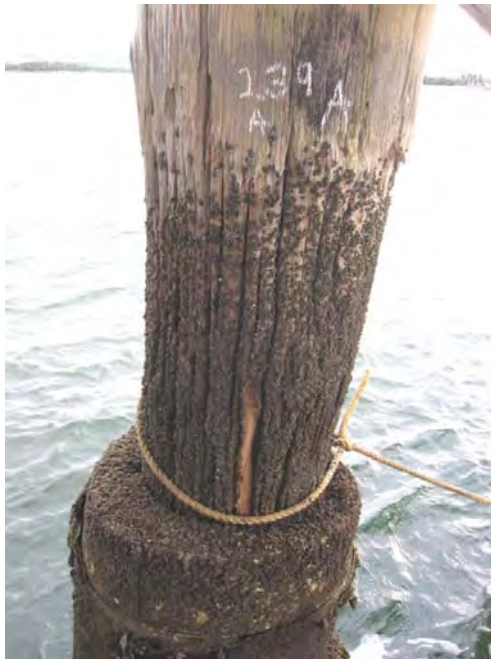
Figure 13: Pile 239A with concrete collar to about mid-tide, showing fissures 10-15 mm deep due to weathering, marine borer damage mostly absent in tidal zone.
