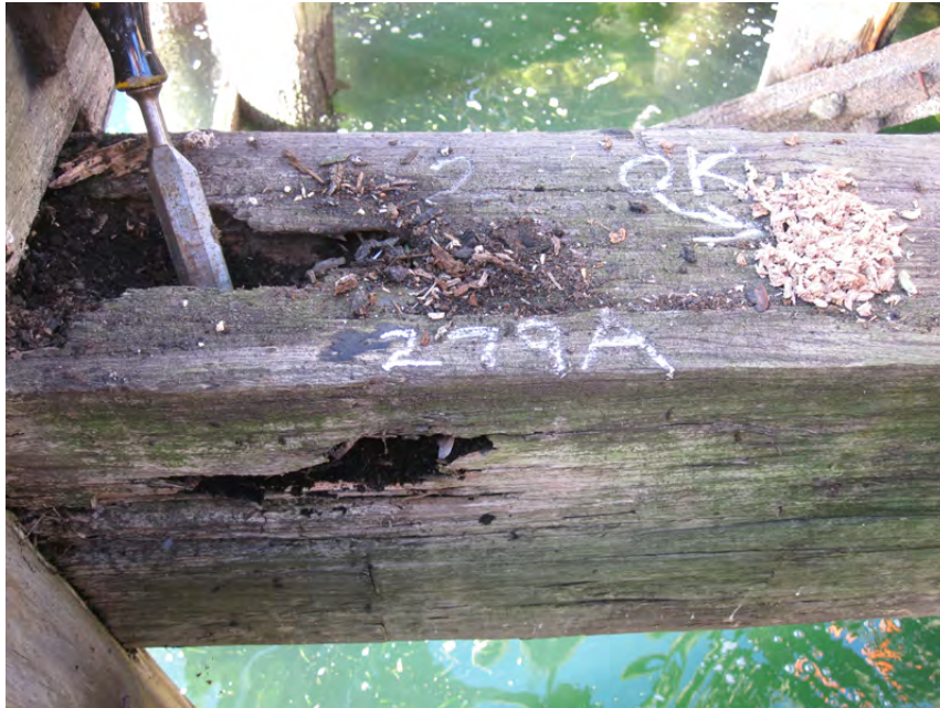
Figure 16: Crosshead 279A showing end with extensive termite damage, and drilled shavings ('OK') further from end from which sound timber begins.
