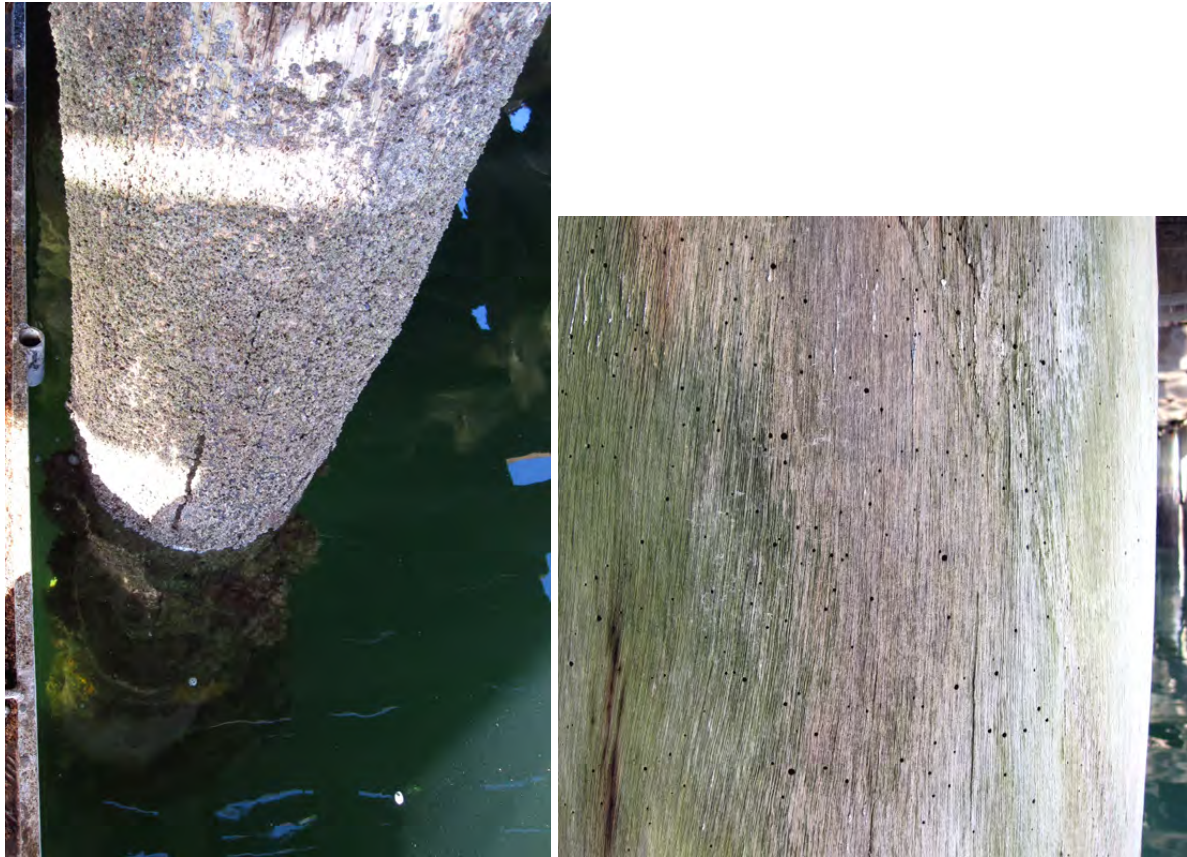
Figure 23: Pile 297B, without necking of heartwood and ~270 mm sound heartwood remaining. Left photo showing heavy Lyctus borer damage to sapwood (not heartwood) above the tidal zone.
