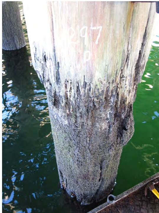
Figure 25: Pile 297D, with several cavities at low tide and 30-40 mm teredinid attack, with ~100 mm sound heartwood remaining. Pile unserviceable.
