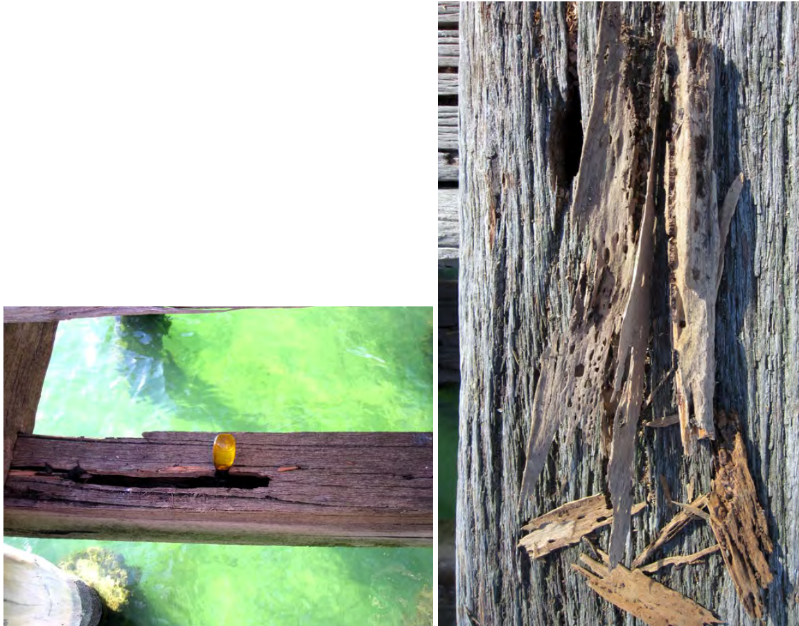
Figure 1: Crosshead hollowed out by termites. Right photo showing 'paper thin' layers of wood pulled from hollow, which is typical of termite attack.
