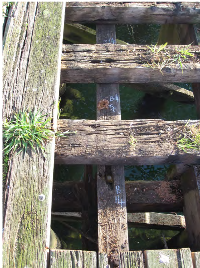
Figure 19: Longitudinal beam 14 near crosshead 278 with severe termite attack one end for approximately 2000 mm length.
