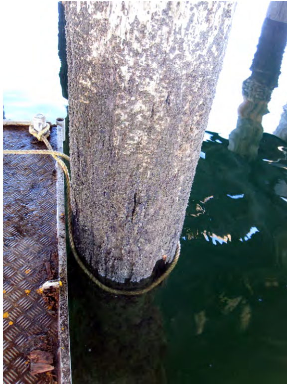
Figure 24: Pile 297C, with cavity caused by Limnoria (right side near rope), and probably with ~230 mm sound heartwood remaining. Pile in poor condition.
