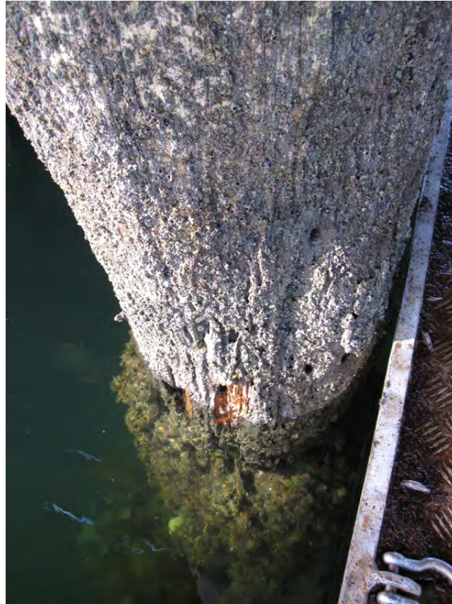
Figure 22: Pile 296B, with ~270 mm sound heartwood remaining. Freshly chiseled region near waterline showing some white calcareous-lined teredinid tunnels.
