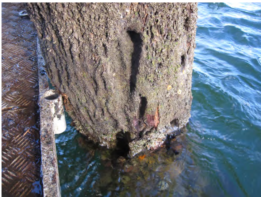
Figure 7: Pile 236A, showing low tide region with several areas eroded by Limnoria to 30 mm deep in north/south faces. Bolt just below waterline in low tide region.
