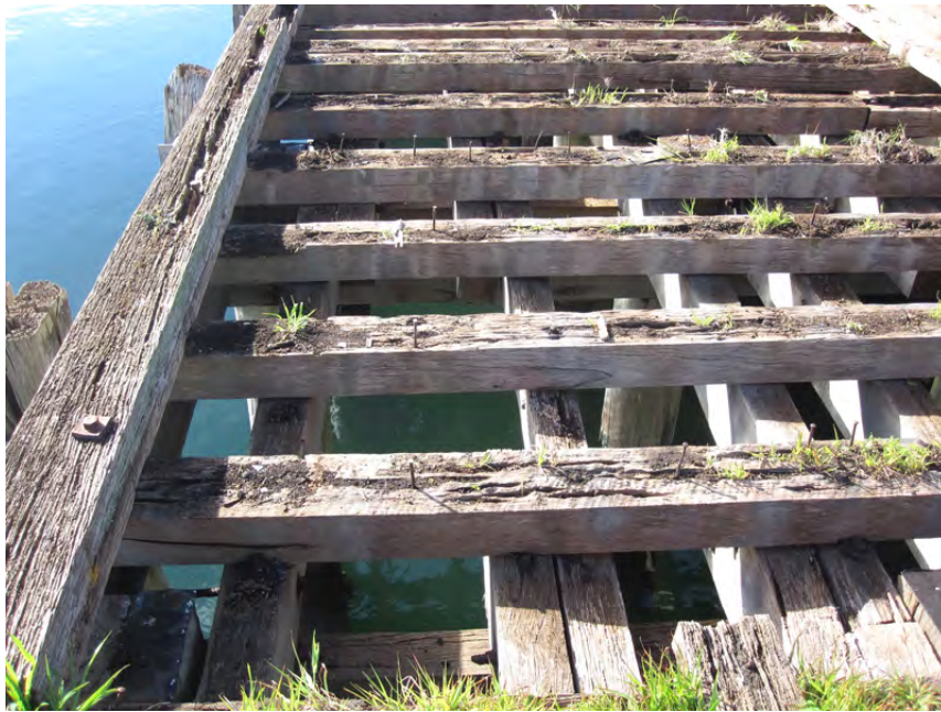
Figure 26: Area 5, decking joists resting on longitudinal beams resting on crossheads.
