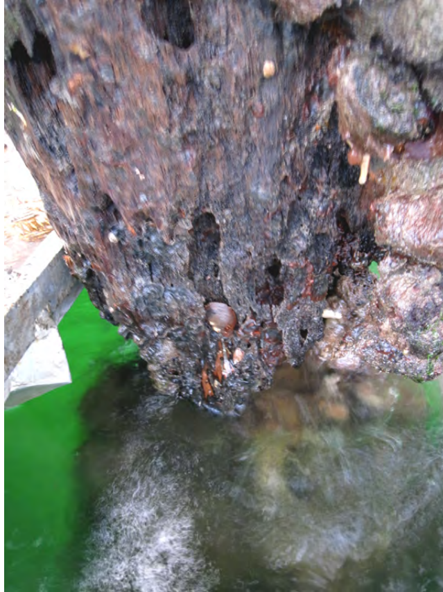
Figure 15: Pile 240B, low tide region showing deep southern cavity at water line on right (below clump of fouling), and shallower cavity on left side. Pile in poor condition.
