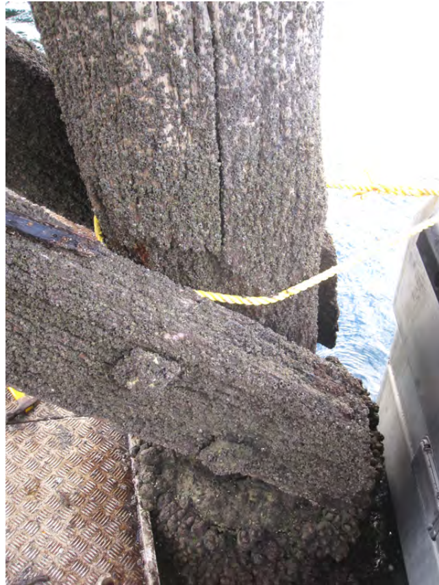
Figure 8: Pile 236B, lower tide region, note pile area near rope notched to fit cross-brace. Concrete collar below cross-brace.
