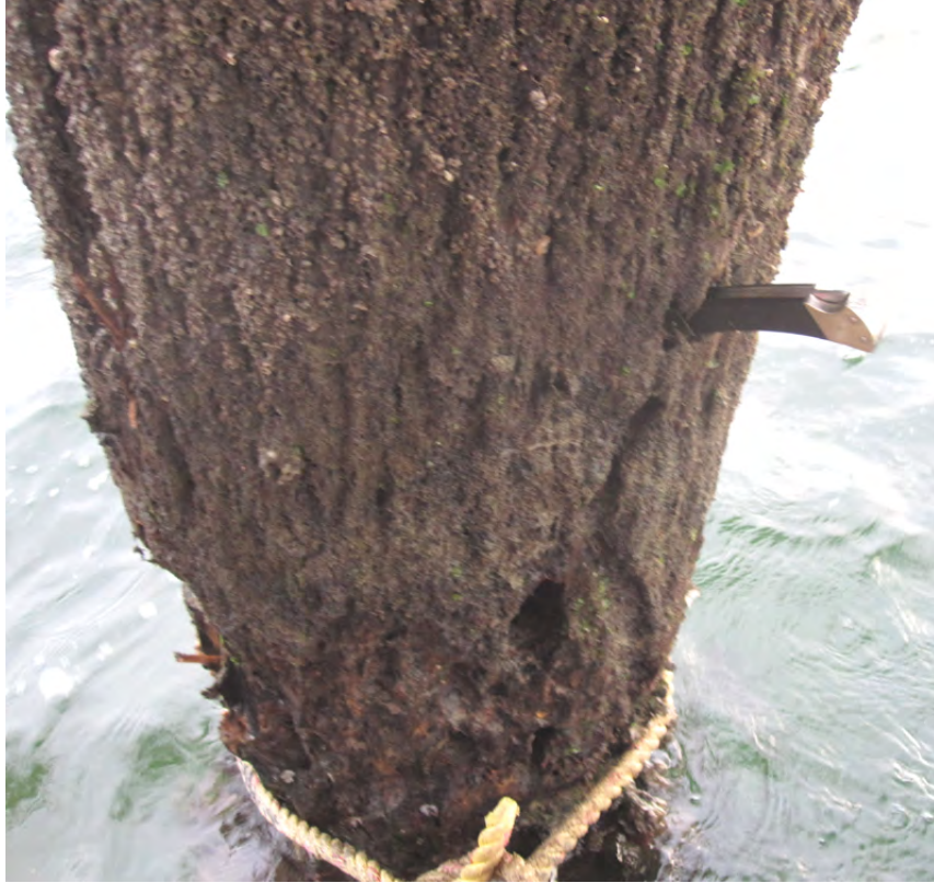
Figure 11: Pile 238A, low tide region showing several 30 mm diameter holes 50-70 mm deep perhaps resulting from old bolt holes or eaten out knots.
