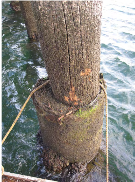
Figure 9: Pile 237A, pile with concrete collar, without active marine borer attack in tidal zone.
