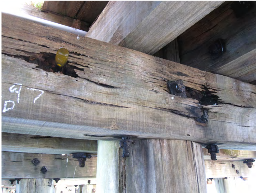
Figure 29: Crosshead above 297 row of piles, heavily attacked by termites (note chisel pushed through timber).
