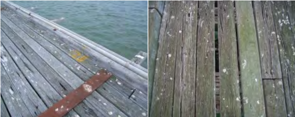
Figures F7-8: Current state of Jetty Structure
