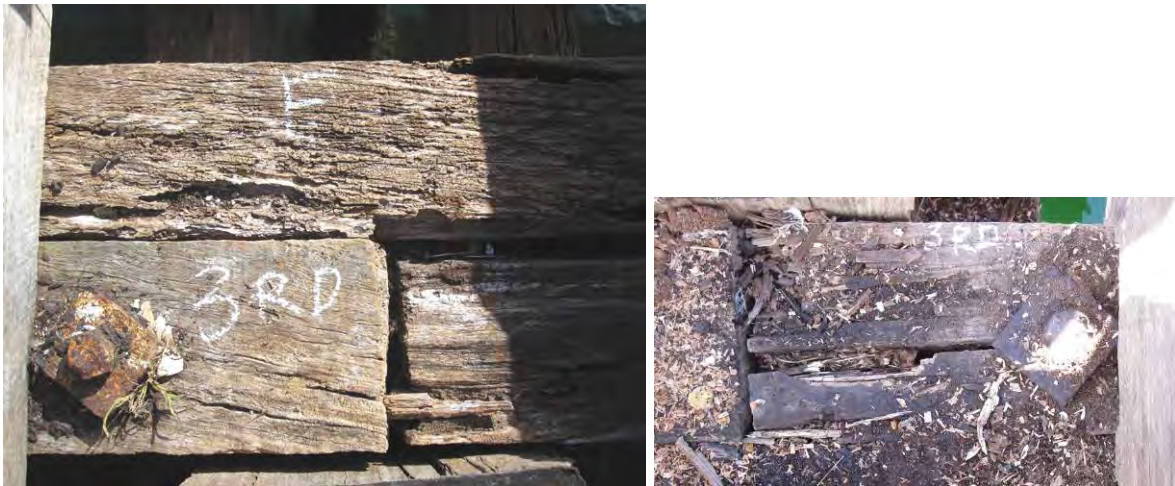
Figure 30: Longitudinal beams, '3rd' shows southern beam in good condition, joining northern beam to right with 20 mm decay on top surface. 'F' is fish beam with up to 60 mm decay on inner face adjacent to other timbers. Right photo shows northern end of northern beam with 100 mm white rot to 250 mm from end.
