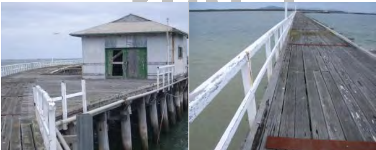
Figures F12-13: Timber handrails
