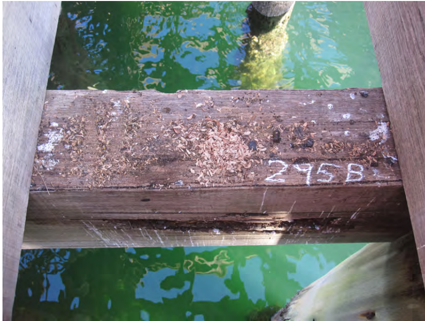
Figure 27: Crosshead above 295B pile, showing damaged pith area (closest face) on side, drilled shavings on top face indicate remaining heartwood in good condition.
