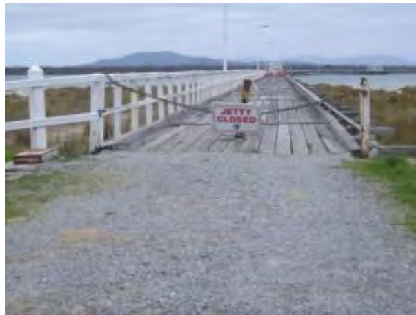
Figure F1: Port Welshpool Long Jetty
