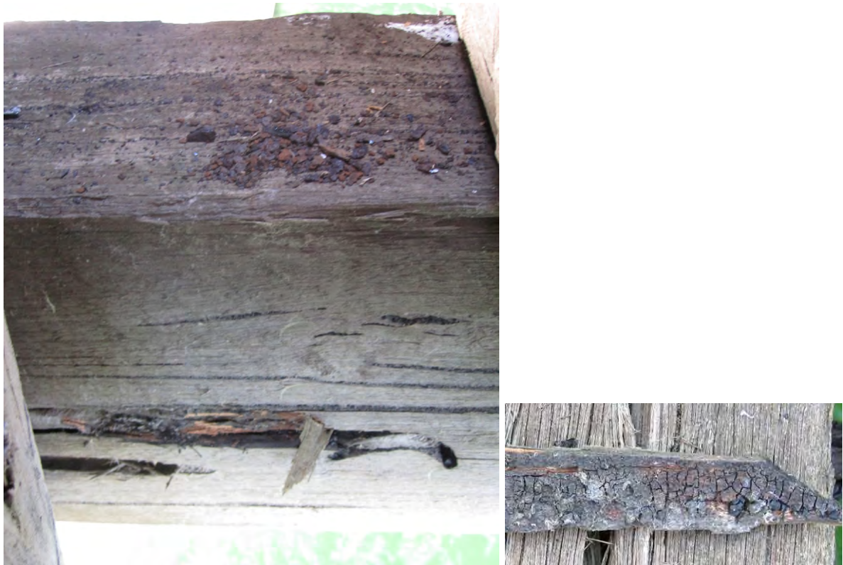
Figure 2: Side of crosshead with 10-20 mm patch of damage from kino and pith, of minor concern. Right photo shows dried kino on removed piece.
