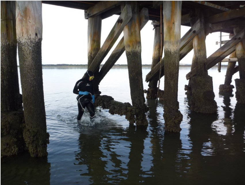
Diver inspecting Bents 201-210 at dead low tide.
