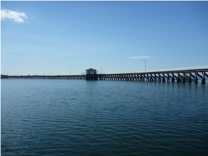
Piles Inspected: Bent 142- 251
