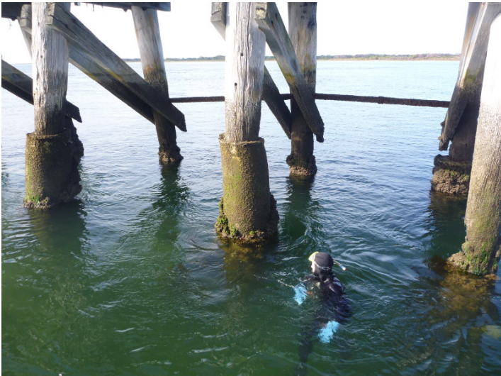
Typical concrete Repairs Trestle pile section
