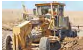
Road Construction & Maintenance
