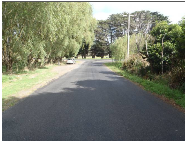
Figure 14: Sommers Crescent View North-West to Jumbunna Road
