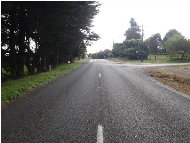
Figure 7: Jumbunna Road & Sommers Crescent Intersection – View North-East
