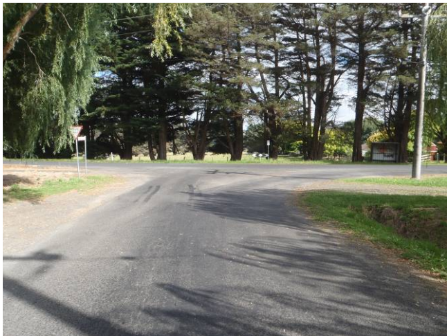
Figure 13: Jumbunna Road & Sommers Crescent Intersection – View North-West
