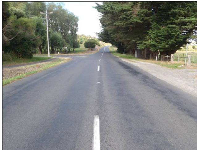
Figure 8: Jumbunna Road & Sommers Crescent Intersection – View South-West
