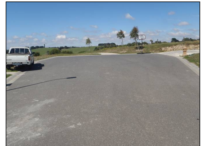
Figure 15: Prudence Close at South End – View South
