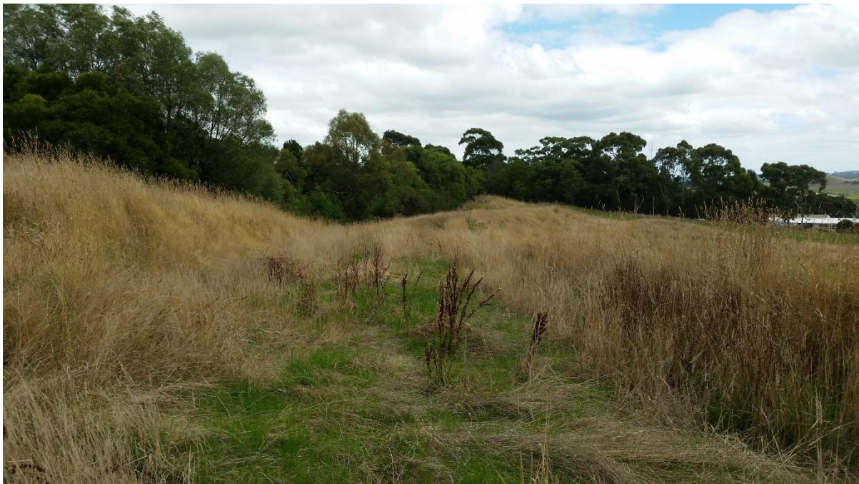
Photograph 2: The location of the former railway embankment is still clearly evident today. A cut and fill approach was used to construct the embankment, thus it is expected that material used to build up sections of the former railway embankment was from onsite and not imported materials.
