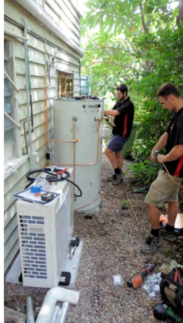
Installation of a heat pump hot water system. Image: Whywait Plumbing Services www.whywait.com.au
