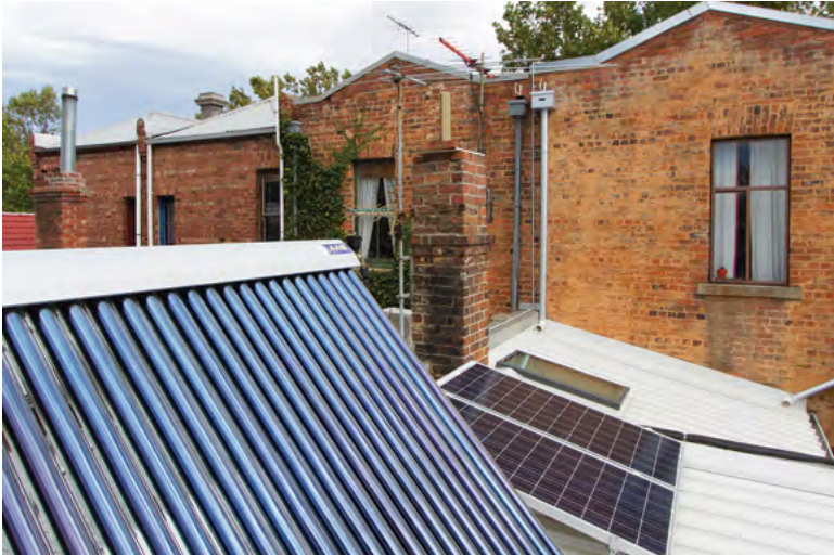
The heat from the tubes is transferred to the water via a copper heat pipe. Image Nic Granleese.
