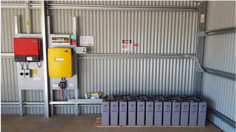
A typical AC-coupled hybrid system. The battery bank is on the right, the yellow box is the inverter/charger and the red box is the grid-interactive inverter. Image: Off Grid Energy Australia.
