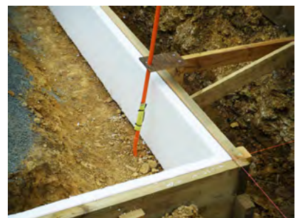
↑ The slab insulation, before pouring of the slab.
