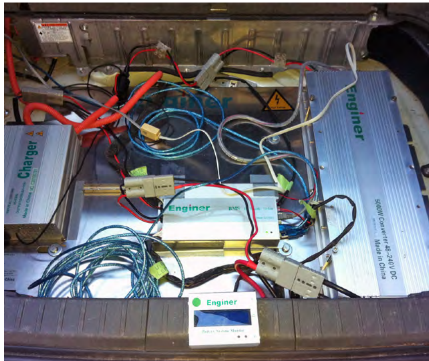
↑ This is the plug-in Prius conversion kit in the Prius's boot. On the left is the 48 volt mains battery charger and on the right is the 48 to 240 volt DC-DC converter, which takes power from the add-on battery (the large silver box underneath everything else) and steps it up to match the Prius's system voltage. Alan's home power system runs from the 48V battery. The small box in the middle is the battery's management system.
