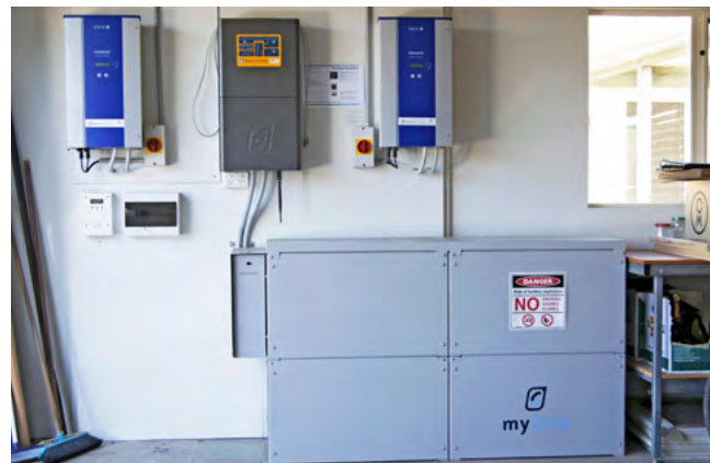
↑ The neat installation of the Selectronic myGrid system using Sonnenschein sealed lead-acid batteries and an SP-Pro inverter-charger.
