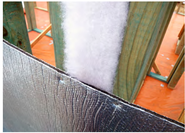
↑ Foil/foam composite insulation and thermal breaks improve energy efficiency.
