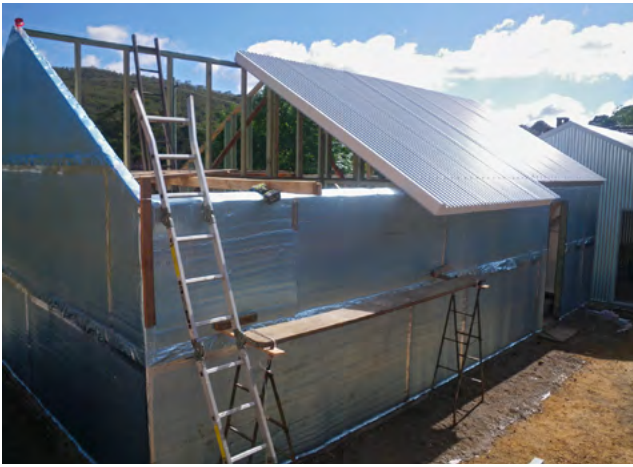
↑ The roof consists of corrugated-iron-clad SIPs, making for a quick installation.
