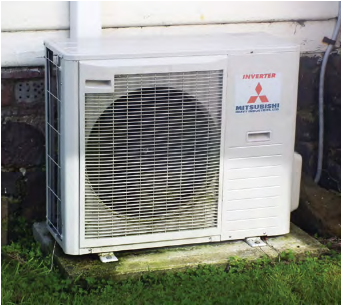
↑ The compressor unit of a split system. Mounting it in full sun with a deciduous tree or eaves for summer shade can improve system efficiency.
