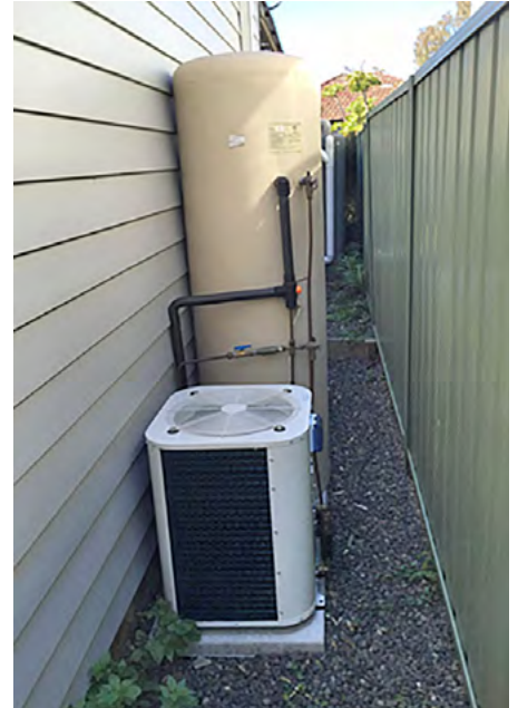
↑ Here is what our system looks like, with the heat pump in the foreground and the tank behind it.
