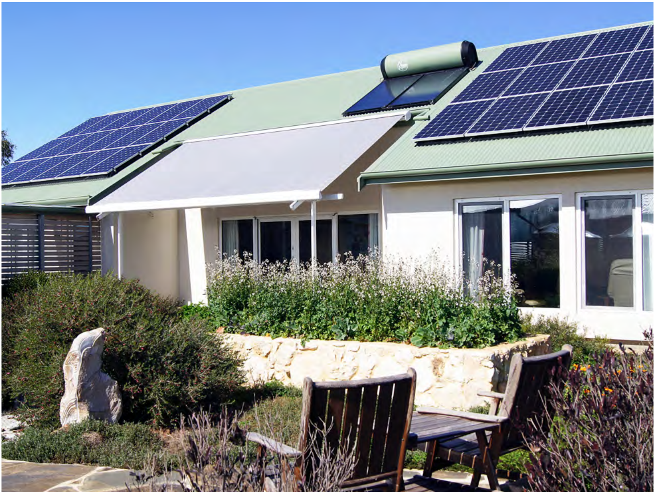
↑ John and Elizabeth's home with almost 10 kW of PV and PV-boosted solar hot water. The shade in front of the solar hot water system is retractable for winter warming of the internal thermal mass.
