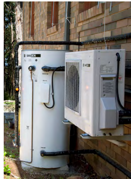
↑ Your existing electric hot water service, either resistive element or heat pump, can provide energy storage at much lower cost than a battery.
