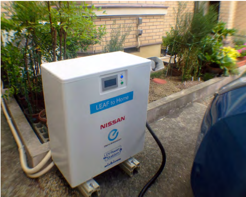
← Nissan's Leaf-to-Home bi-directional charging system is capable of supplying up to 6kW of AC power drawn from the Leaf's 24kWh battery. This system is currently available for Japanese EV drivers at a cost of around $5000 before a government rebate (which effectively halves the purchase price).
