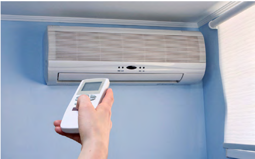
← Split system reverse-cycle air conditioners are compact and simple to operate and modern units generally have high operating efficiencies.
