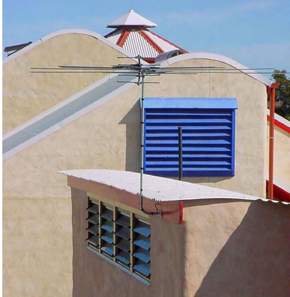
↑ Four kinds of controllable ventilation at Christie Walk use heat rising up stairwells to high level outlets. Clockwise from top left: openable skylight; vents in the peak of a roof; vents from attic; and openable louvres. Photo by Paul Downton
