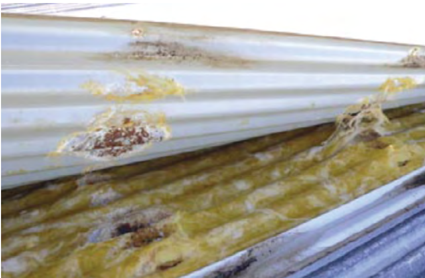
↑ Different climates require different strategies to avoid condensation problems. Here, in a tropical environment, moisture has caused damage to roofing and insulation due to the absence of an appropriately located vapour barrier. Photo courtesy BlueScope Steel
