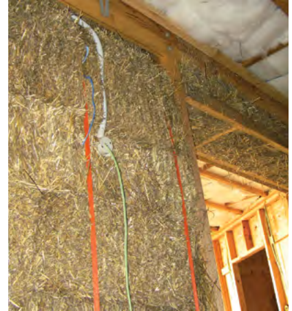
↑ It took a year of construction to make this lovely liveable space. You can see the strawbale walls before the lime render, and after (next page, top). On the north-facing windows, both inside and outside shades keep out the summer sun.
