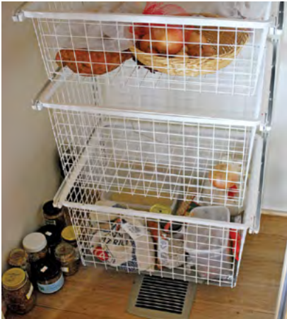
↑ This cool cupboard is kept at a lower temperature, around 16°C in summer and 12°C in winter, with air drawn from an underground tube.
