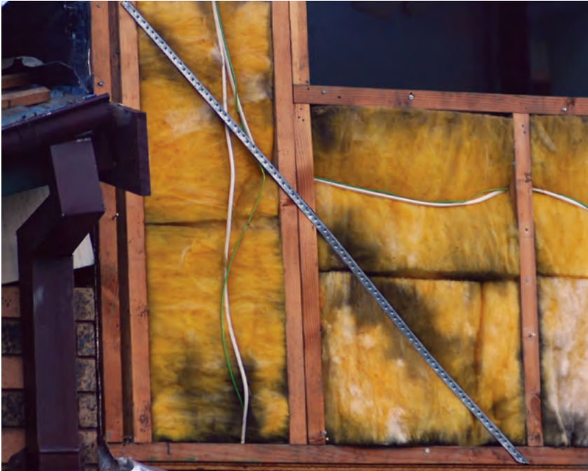
↑ When a frame is filled with bulk insulation and wrapped externally with insufficiently breathable sarking, there is a high risk of condensation forming on the inside of the wrap during winter. This can lead to loss of insulation effectiveness, mould growth and structural damage. Photo courtesy Andy Russell
