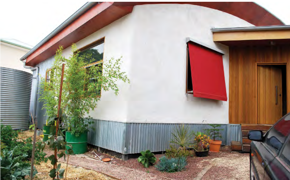
↑ At the front of the house you can see the external shades, rainwater tank, rendered walls and the airlock entry to the right. The driveway gravel is made from crushed, reused concrete and bricks.
