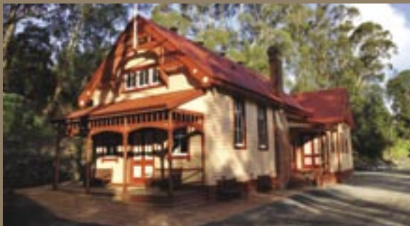
Restored building in Coal Creek Community Park
