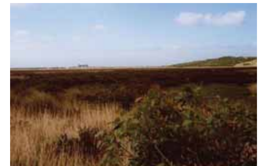
Sewage Treatment Plant: Visible against the skyline from miles away.
