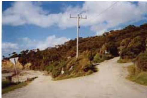
Terminus of Bayside Drive, Waratah Bay: This area is neglected and degraded and gives no sense of arrival.
