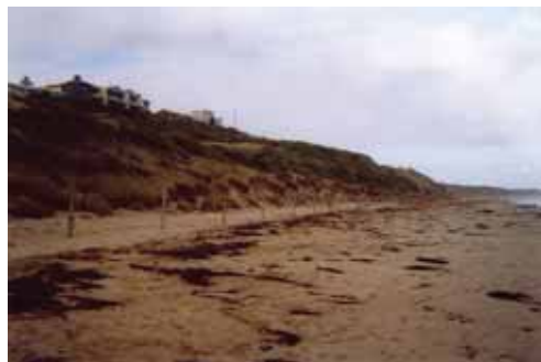
Cliff top houses at Ocean Grove.
