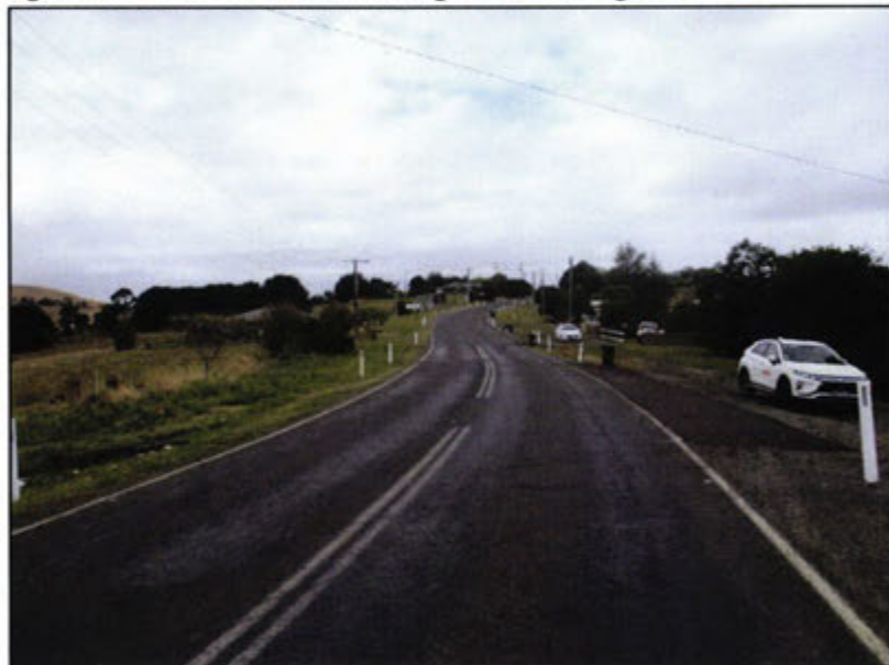
Figure 2.5: View of Korumburra-Warragul Road Looking Southeast
