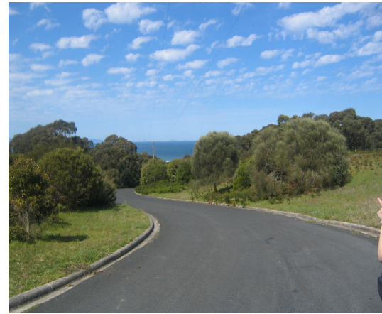
Photo 5. Road connecting upper and lower sections of Waratah Bay.
