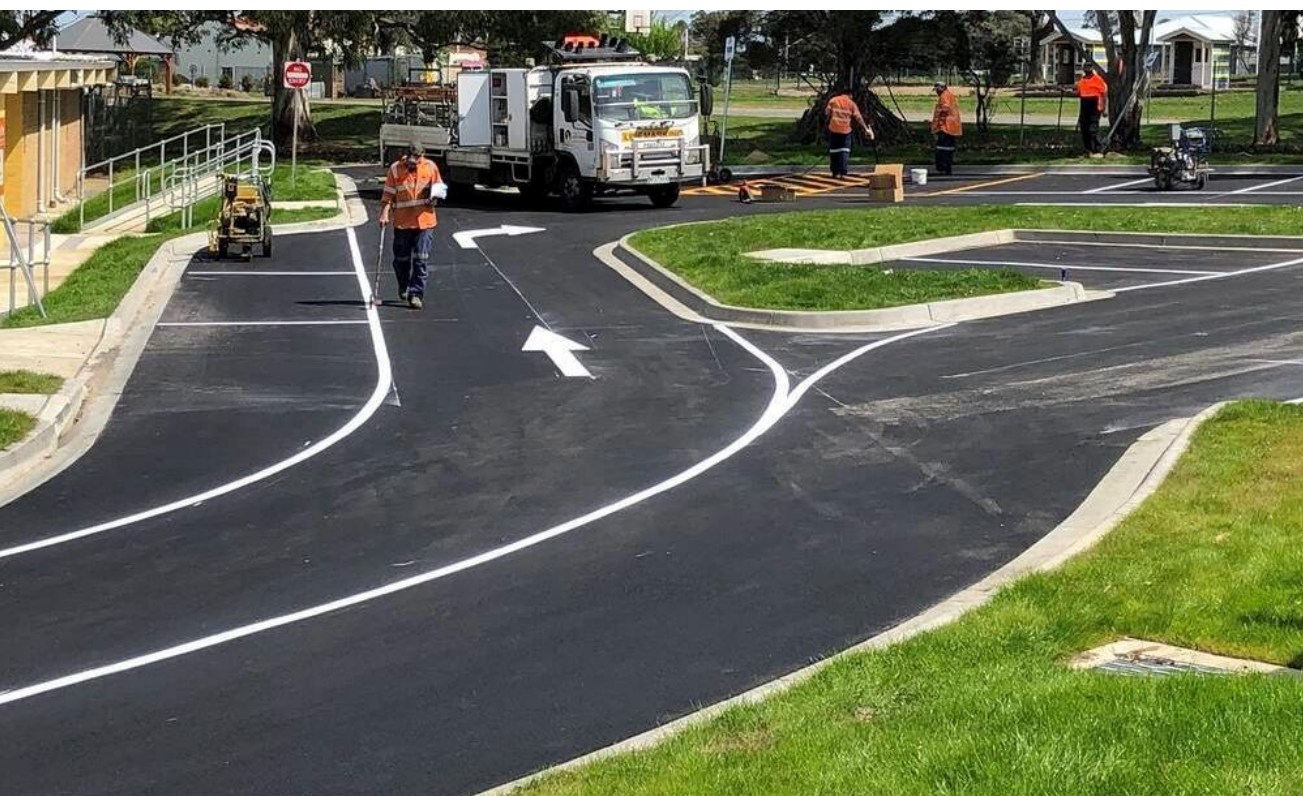
Council's Road Crew
