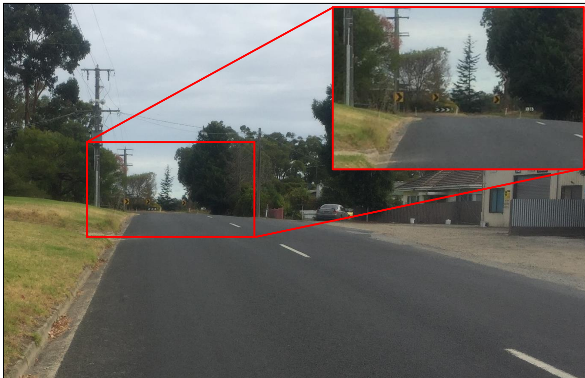
Figure 15: Southern Sight Line from Southern Access Road on Davis Street
