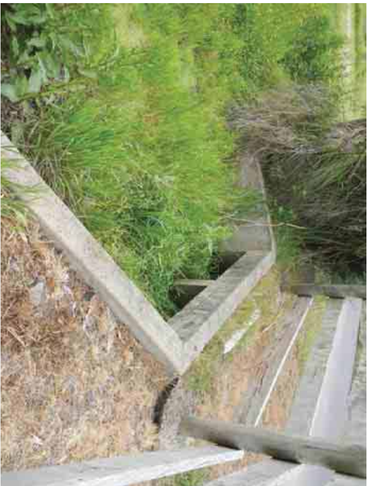
Figure 3.5 View north to the inlet of the 2 no. 1200 mm wide by 600 mm high box culverts located under Follett Drive
