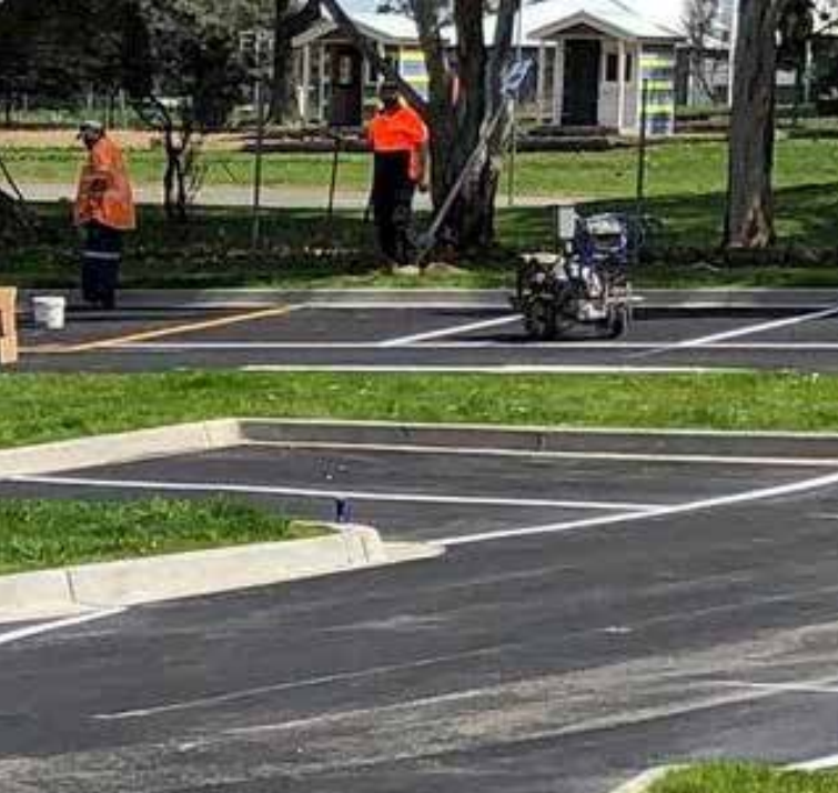
Road Works Crew
