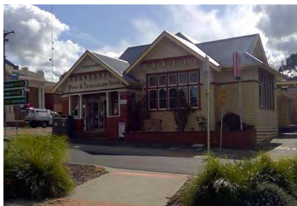
Leongatha Post & Telegraph Office - Heritage Overlay 71
