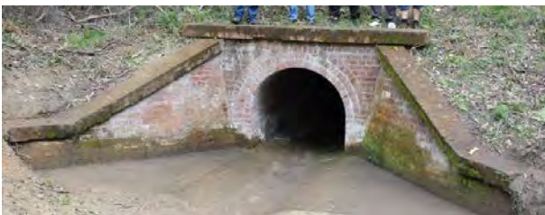
Railway Culvert Mirboo North - no heritage protection
