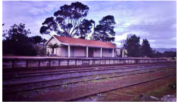
Foster Railway Station - no heritage protection (Photo Credit: Australian Rail Maps )
