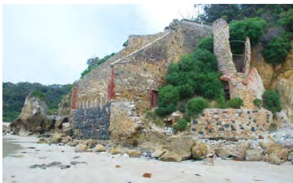
Walkerville Lime Kilns - Heritage Overlay 129
