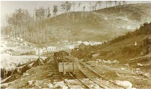
Coal mining in Outtrim (Photo Credit: Leongatha & District Historical Society )
