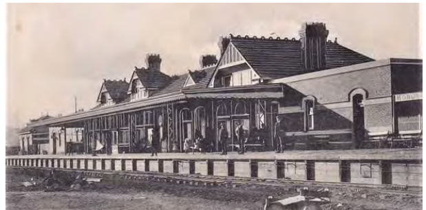
Korumburra Railway Station - Heritage Overlay 18 (Photo Credit: Korumburra Community Development & Action Inc )
