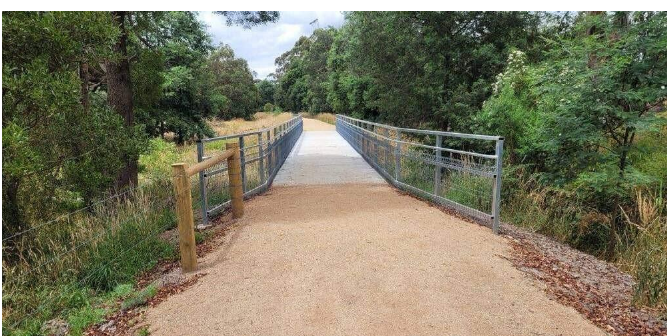
Great Southern Rail Trail
