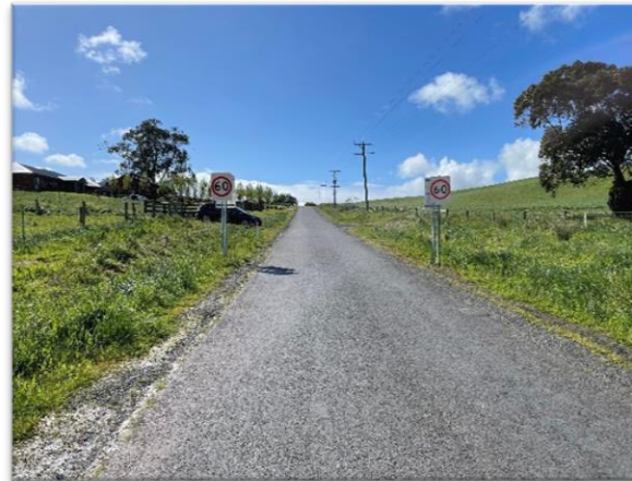
Figure 2.4: Berrys Creek Road, looking east from the site's western boundary
