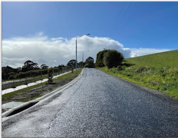
Figure 2.3: Bena Road, looking east from Mountain Ash Drive
