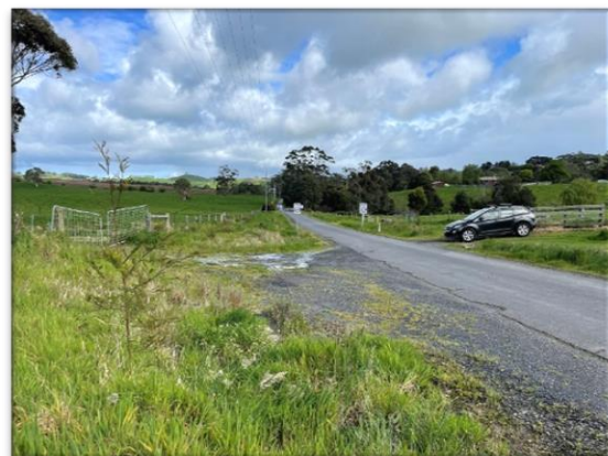
Figure 5.8: Available SISD looking west from the proposed Western Access Point
