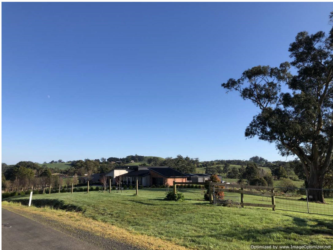
Photo 6 – Existing residences on the north side of Bena Road
