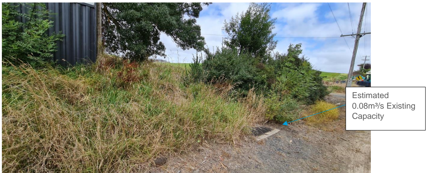
Figure 28. Existing Grated discharge at NE Corner
