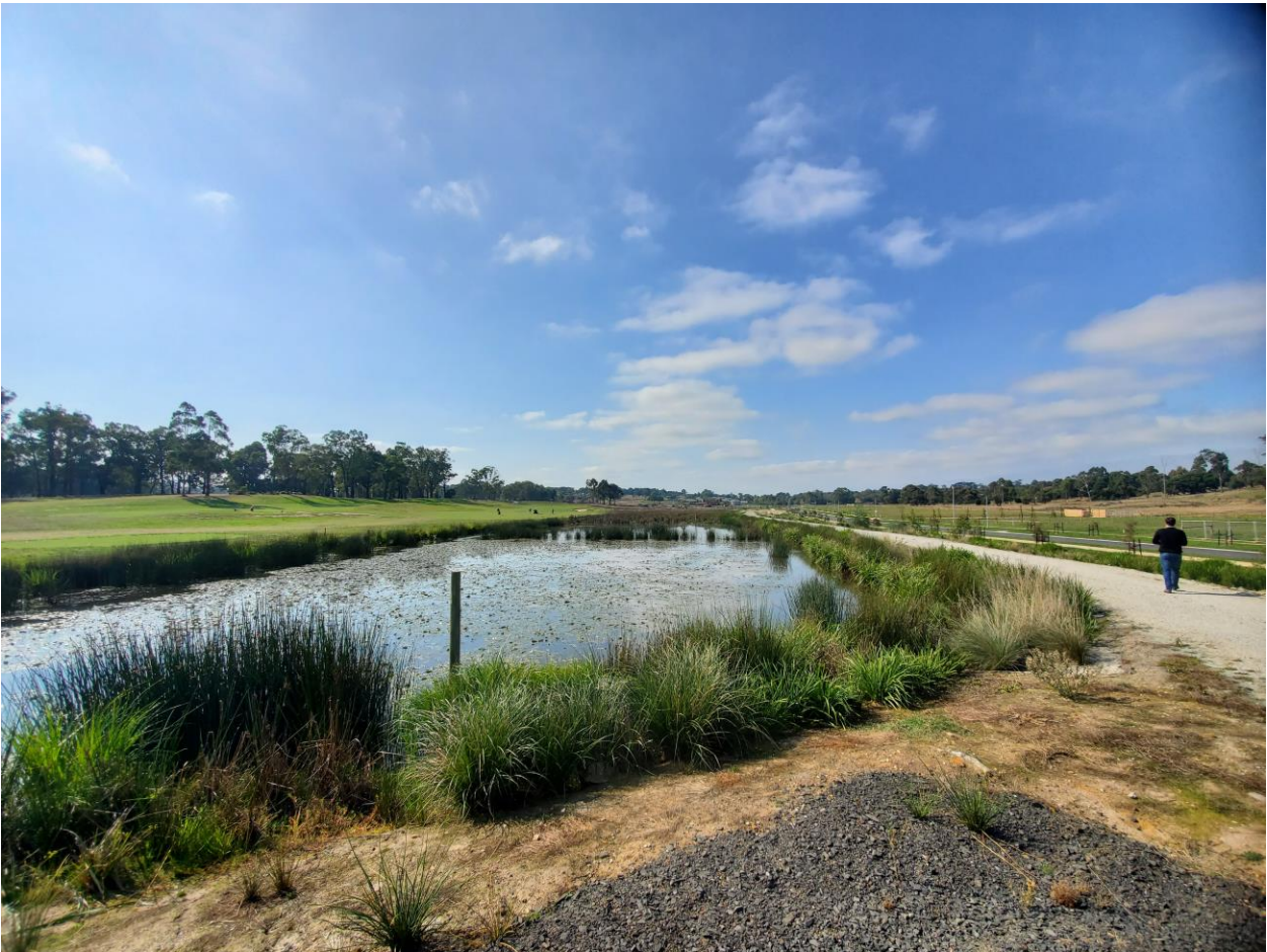
Figure 46. Drouin Wetland and Bypass Channel
