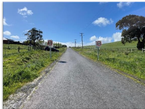
Figure 2.4: Bena Road, looking east from the site's western boundary towards Mountain Ash Drive
