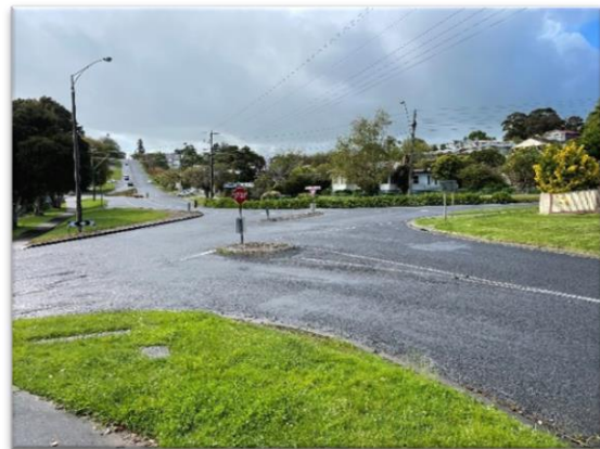
Figure 2.6: Bena Rd/ George St Intersection looking east towards Radovick St
