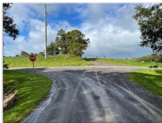
Figure 2.7: Bena Road/ Whitelaw Road Intersection, looking south
