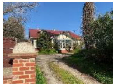
Figure 54. Interwar bungalow at 325 High Street
