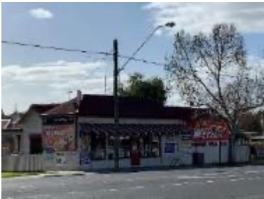
Figure 49. Store and residence on corner Maple and High streets
