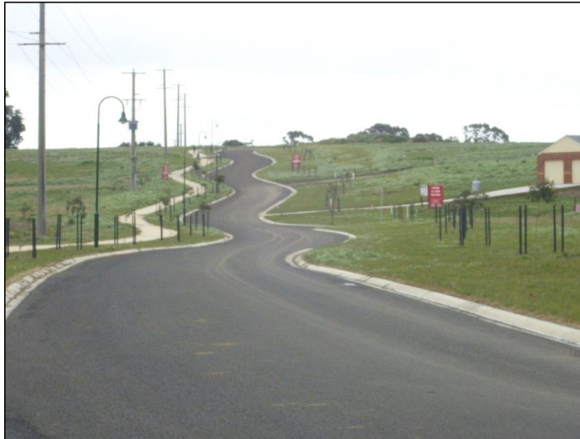
Photo 5: Tarwin Ridge Road, looking north
