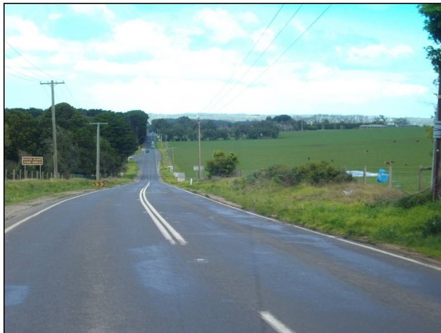
Photo 2: South Gippsland Highway, between Parr Street and Simons Lane, looking south
