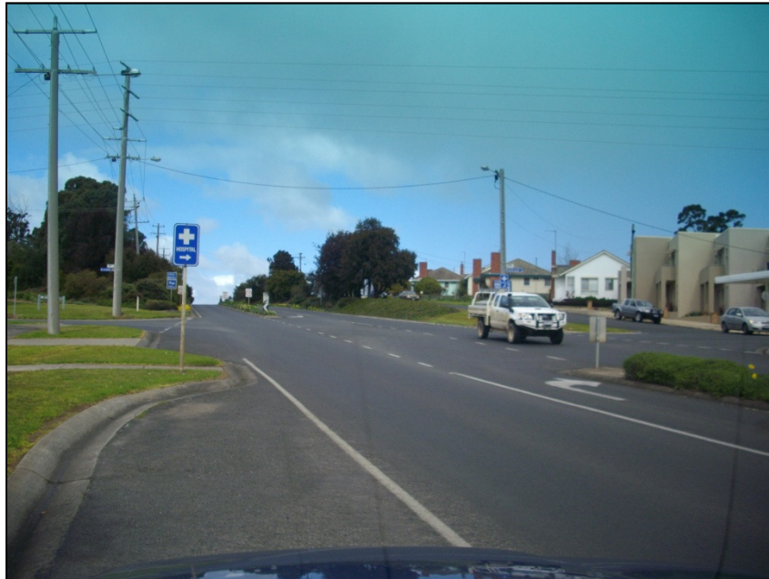
Photo 1: South Gippsland Highway / Parr Street intersection, looking south
