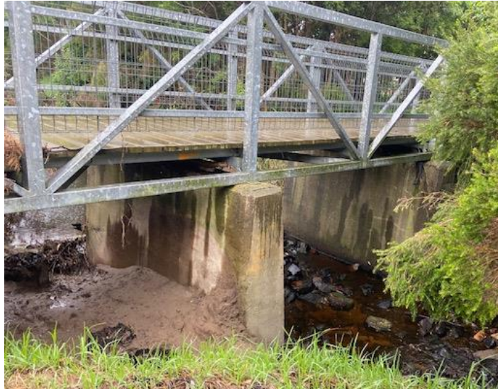
c) Rail Trail Creek Crossing
