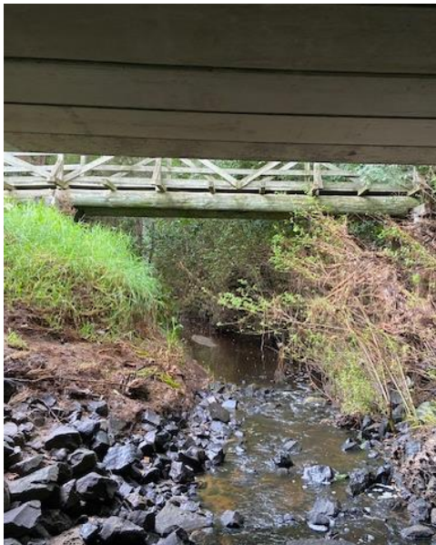
b) Pedestrian Bridge adjacent to Highway
