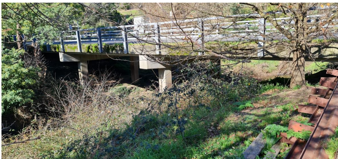
Figure 2. Existing Bridge Structure
