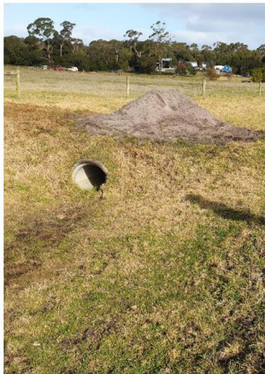
Figure A 3 Cross culvert pipe from site inspection (south/downstream end)
