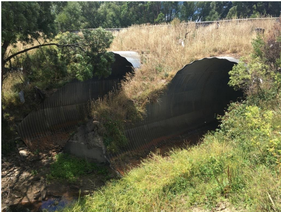
Figure 9 Photo of Falls Road Culverts (taken during site visit)
