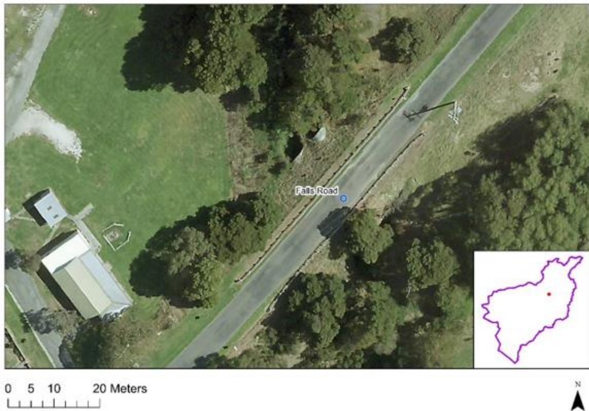
Figure 8 Imagery of Falls Road Culvert
