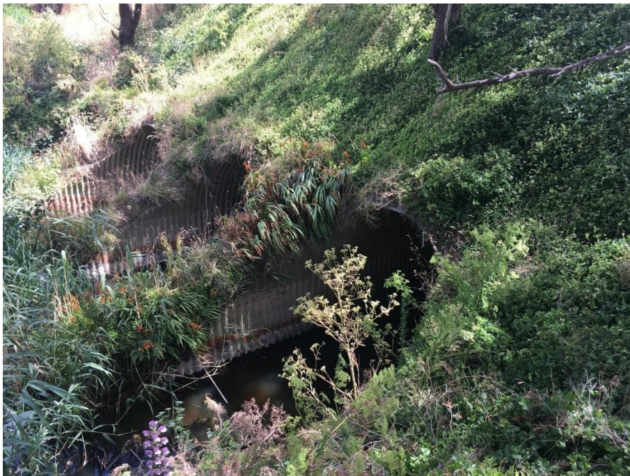
Figure 12 Meeniyah-Promontory Rail-Trail Culverts
